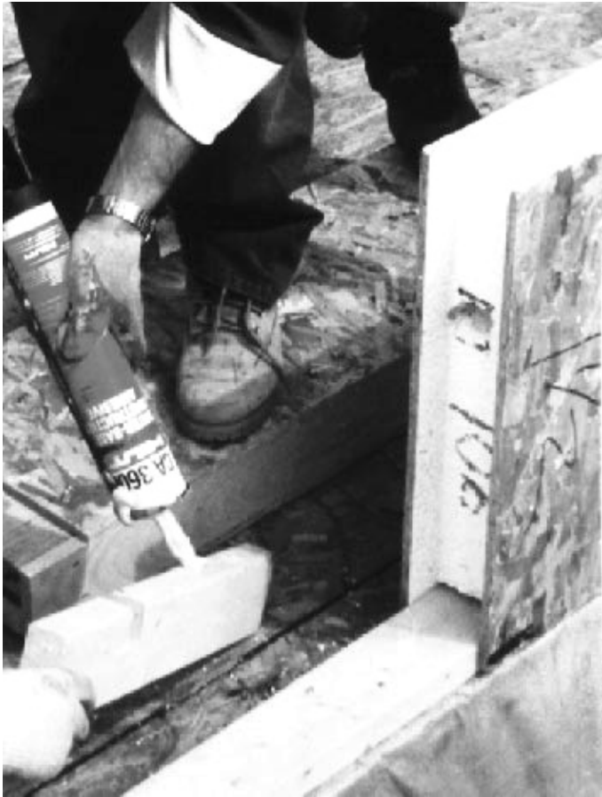
Figure 15.5 SIP adhesive/sealant. (R-Control Building Systems)
