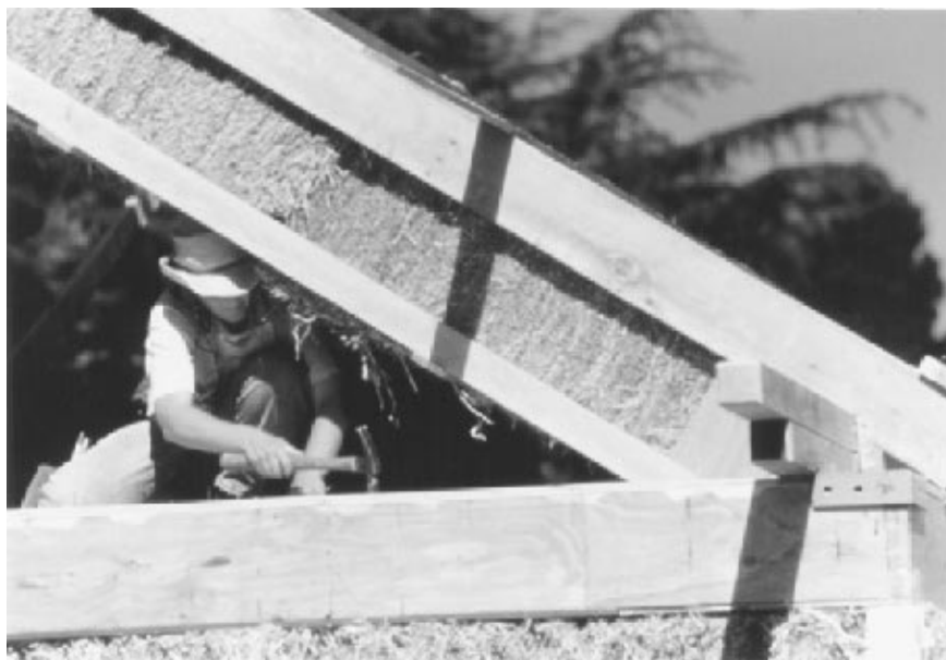
Figure 15.34 Roof detail. (Daniel Smith & Associates, Architects)
