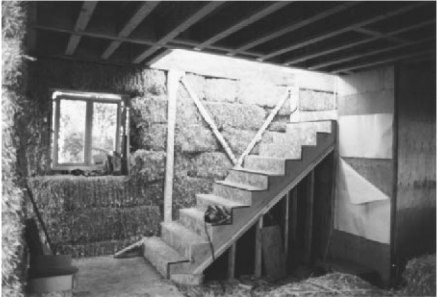
Figure 15.27 Berkeley cottage interior. (Daniel Smith & Associates Architects)
