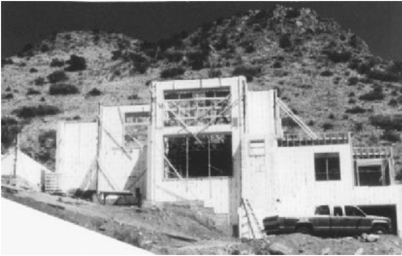
Figure 15.18 Residence during construction. ( American Polysteel, Inc. )
