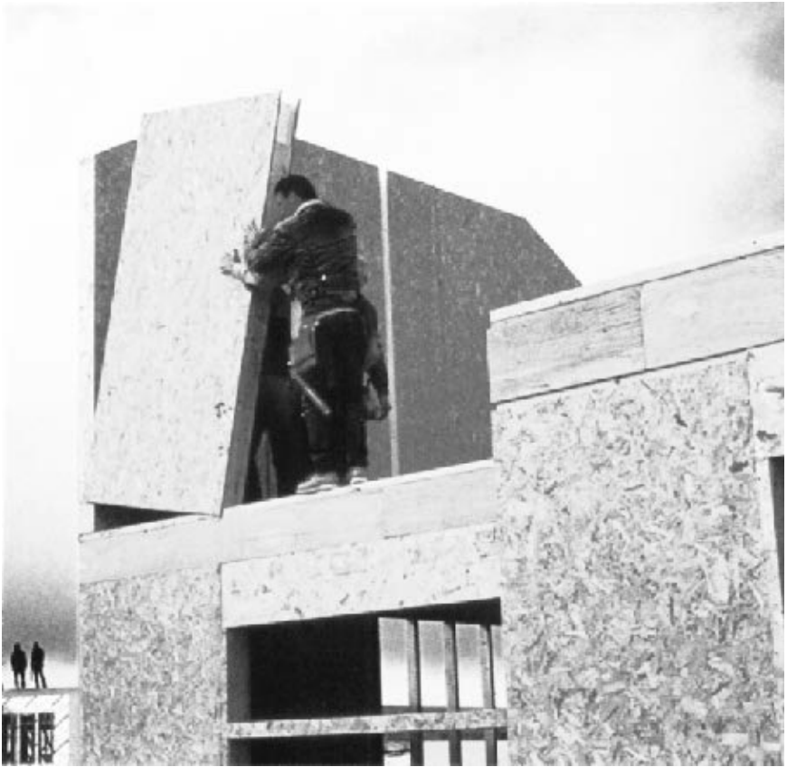
Figure 15.2 SIP wall panel. ( R-Control Building Systems )
