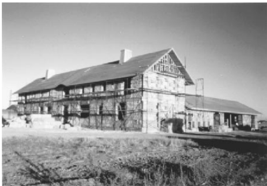
Figure 15.28 Two-story Escalon house under construction. ( Daniel Smith & Associates Architects )
