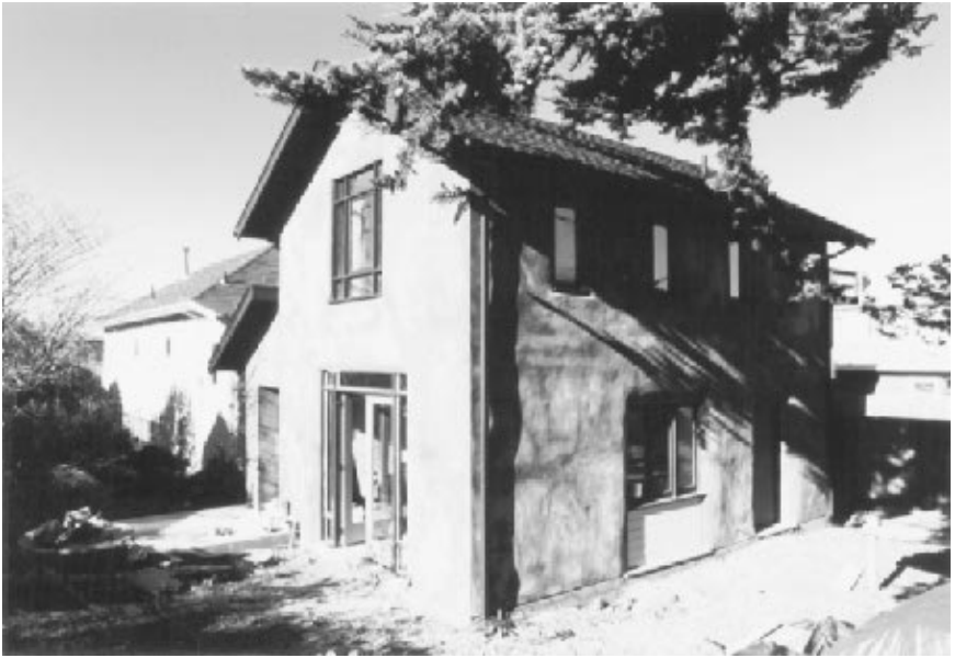
Figure 15.37 Berkeley cottage after stucco. ( Daniel Smith & Associates, Architects )
