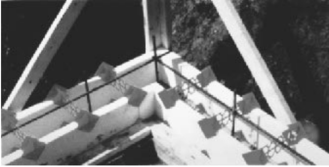
Figure 15.16 Plank system. ( R-Control Building Systems )
