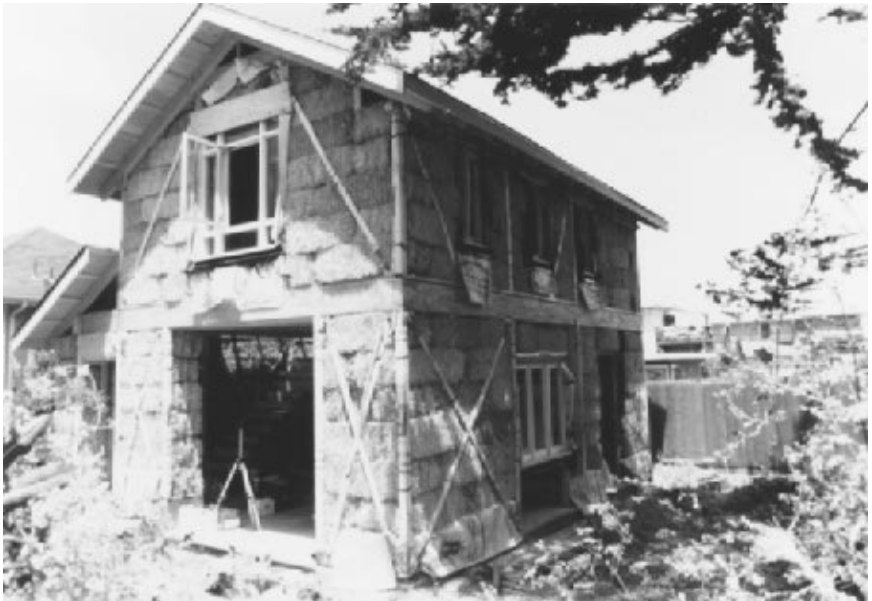
Figure 15.36 Berkeley cottage under construction. ( Daniel Smith & Associates, Architects )
