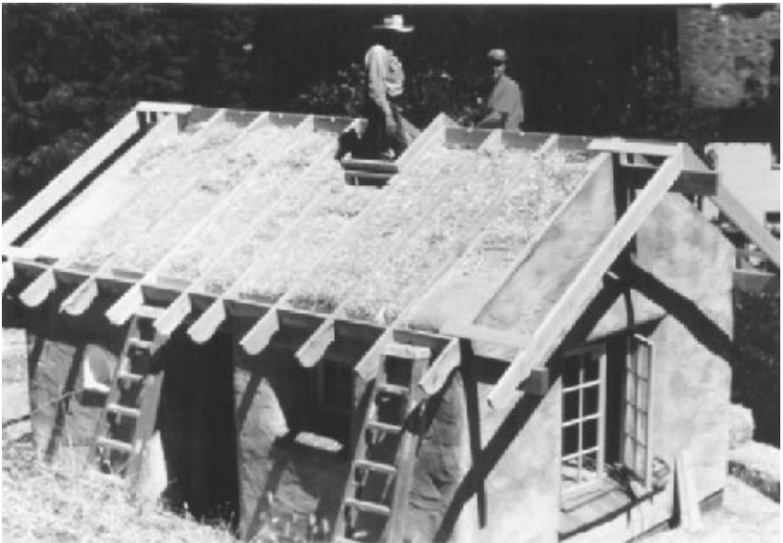
Figure 15.35 Straw-bale roof. (Daniel Smith & Associates, Architects)
