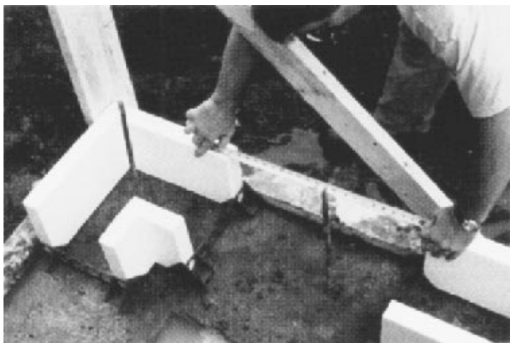
Figure 15.21 Installation of corner units. ( R-Control Building Systems )
