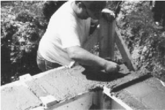
Figure 15.25 Concrete preparation. ( R-Control Building Systems )
