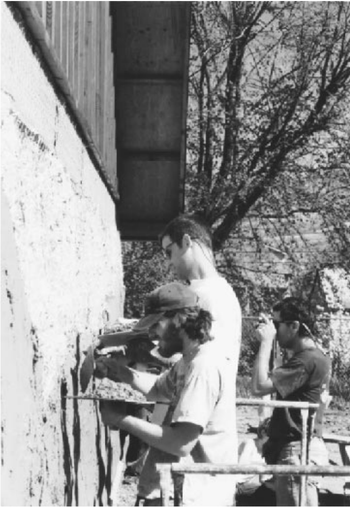
Figure 15.30 Stucco application. ( Harvest Built Homes )
